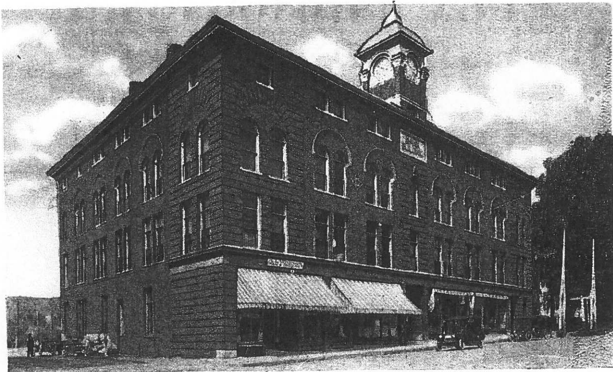
BANK BUILDING. LIVERMORE FALLS ME.
